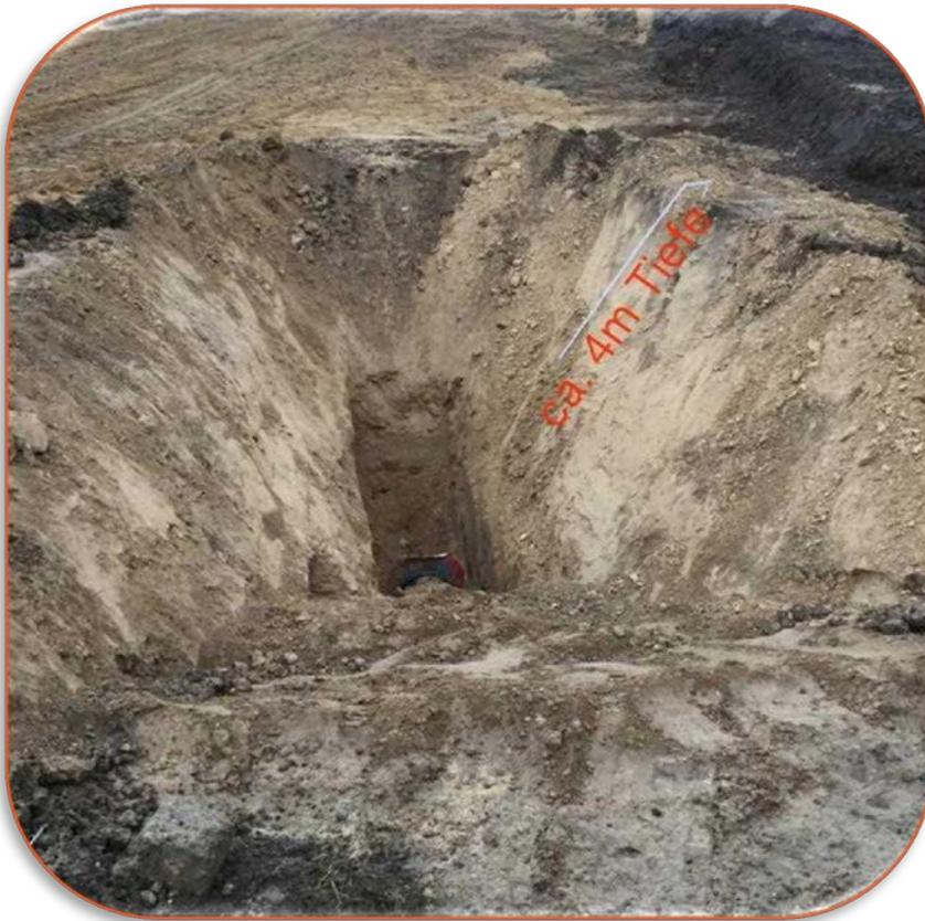
Links: Mangelhafte Baugrubensicherung
